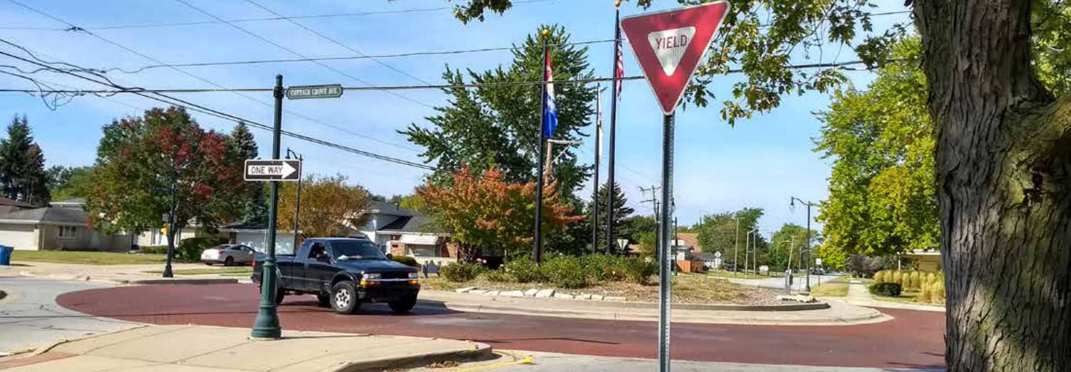
South Holland's well-designed, single-lane roundabout at Cottage Grove Avenue and 166th Street is currently the only roundabout in the south suburbs.
